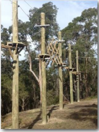
An "Adventurer Trail" built on poles, using a fully continuous belay system of wire rope.
