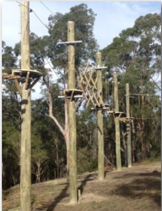
An “Adventurer Trail” built on poles, using a fully continuous belay system of wire rope.
